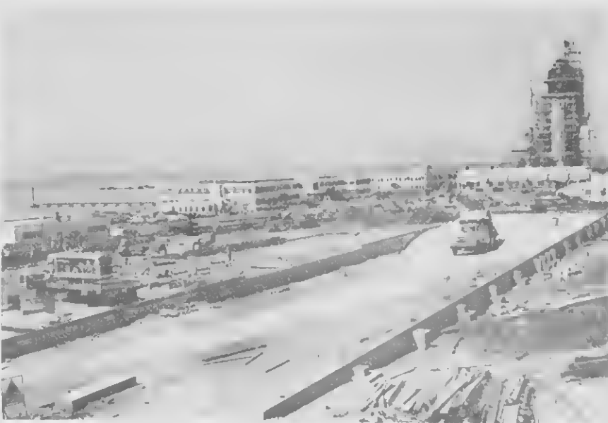
THEN TRUCKLOADS of sand were dumped inside concrete block walls. DESPUES cantidad di truck di santo a worde basha paden di e murayanan.
